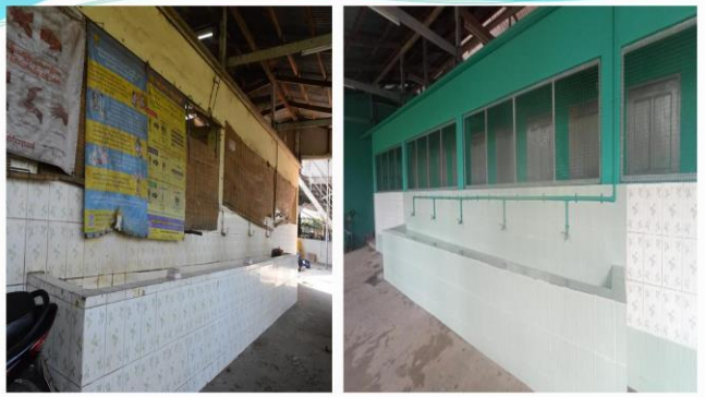
Implementing Activities: Before and After
