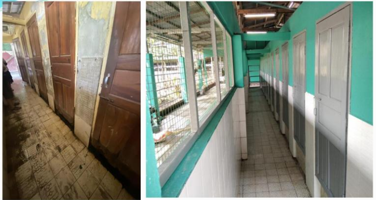
Implementing Activities: Before and After
