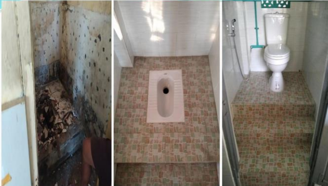
Implementing Activities: Before and After
